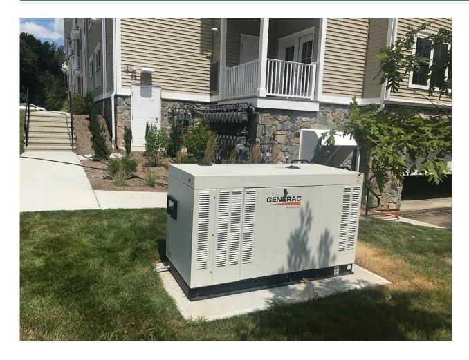
The picture above shows the installation on a concrete pad and close to the natural gas meter that services the common areas.
